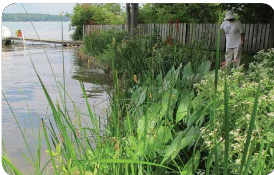
A natural shoreline in its second growing season. Notice wave-breaking coir logs at the far end of the project. Photo: J. Herbert, MSU Extension
