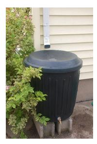
Rain barrels take the downspout disconnect one step further by collecting the rain water that drains off of your roof top. This water can then be used to water your garden and lawn. For every one inch of rain that falls on a catchment area (roof) of 1,000 square feet, you can expect to collect 600 gallons of water using a rain barrel. Watering your garden and lawn takes up 40% of your household water during the summer. Using water from your rain barrel is free!
